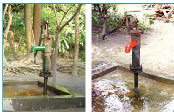
Figure 4. Color labelling of safe (green) and unsafe (red) tubewells in Bangladesh. [Photographs courtesy of Feroze Ahmed, Department of Civil Engineering, Bangladesh University of Engineering & Technology, Dhaka, Bangladesh.]
